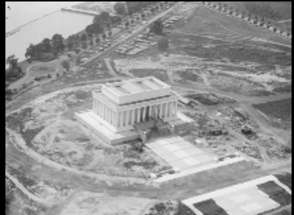
Lincoln Memorial under construction, 1919
